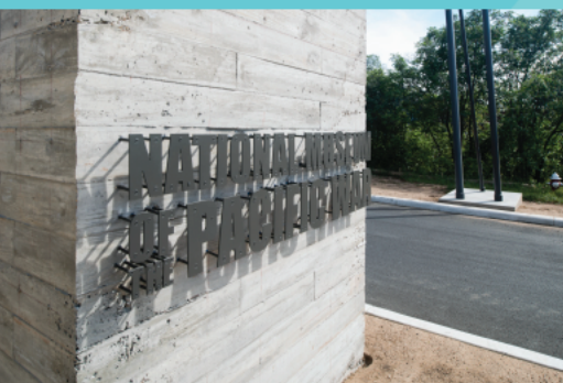
4", 6", 8" AND 9" HIGH WITH 3/16" THICK ALUMINUM LETTERS WITH 3" STAND OFFS
