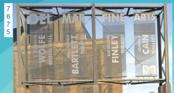
1/8" THICK PRECISION CUT ALUM. MECHANICALLY MOUNTED TO 15" X 5" PERFORATED ALUM. PANELS HELD IN PLACE WITH 1/2" STAINLESS STEEL BOLTS & COMPRESSION SPRINGS
