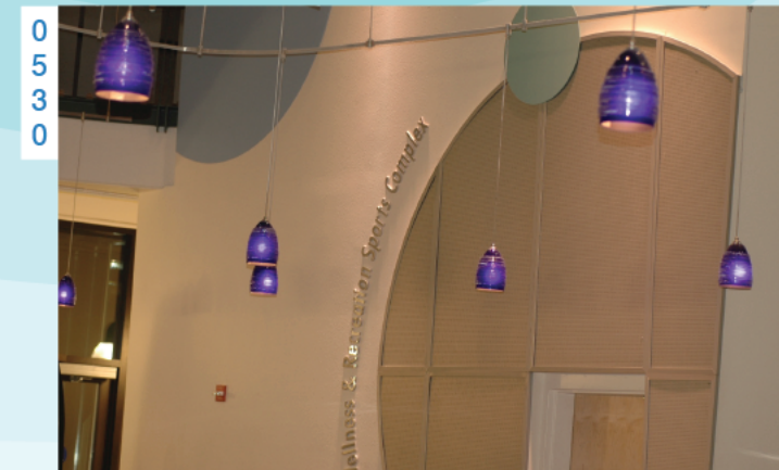
4" HIGH PRECISION CAST ALUMINUM LETTER WITH CUSTOM SHAPED PERFORATED ALUMINUM PANELS WITH ALUMINUM FRAMES
