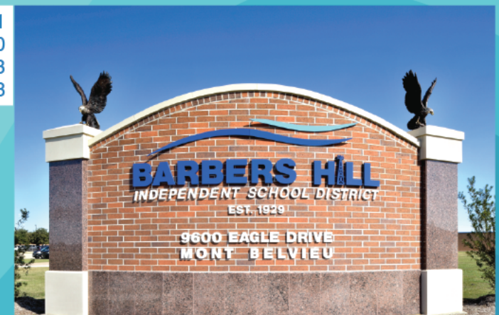
TOTAL LETTER HEIGHT WITH GRAPHIC 6'-1/2" HIGH, CAST ALUMINUM PAINTED FINISH
