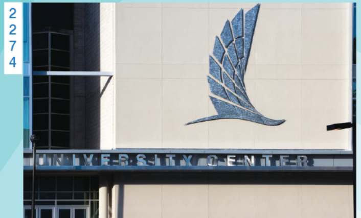
18" HIGH, 3/8" THICK ALUM. WITH RANDOM PATTERN SWIRL FINISH, PROJECTED 4" OFF WALL.
