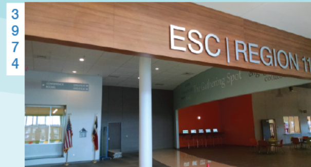
12" SATIN ALUMINUM METAL FACE OVER 1/4" CLEAR ACRYLIC SUBSTRATE
