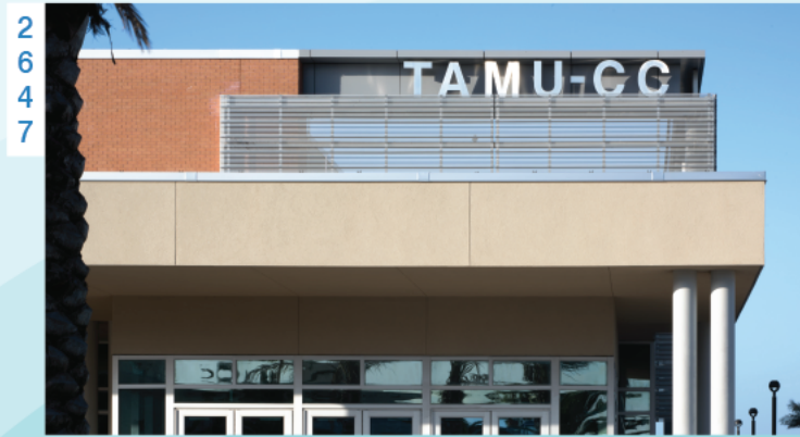
32" HIGH, 4" DEEP STAINLESS STEEL CUSTOM FABRICATED LETTERS
