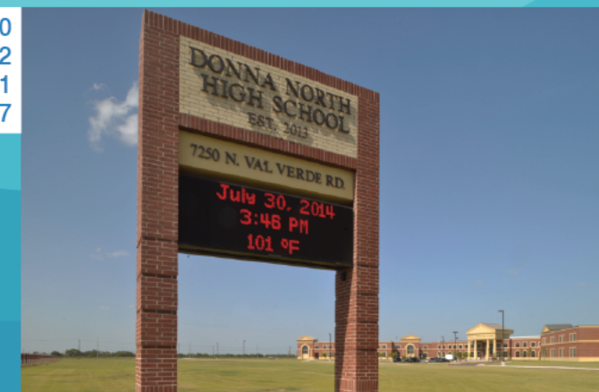
LETTER HEIGHT IS 14" AND 9", CAST ALUMINUM PAINTED FINISH
