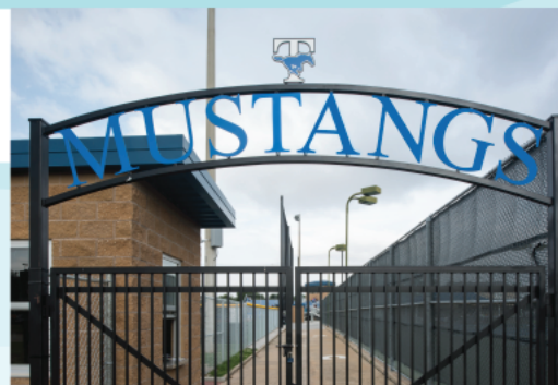
15" HIGH PAINTED ALUMINUM LETTERS AND LOGO, CUSTOM MOUNTING BRACKETS
