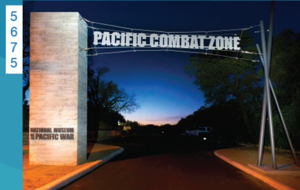
3/16" THICK PRECISION CUT ALUM. MECHANICALLY MOUNTED TO 1-1/2" ROUND PIPE AND SUSPENDED WITH STAINLESS STEEL CABLES AND EYEBOLTS.
